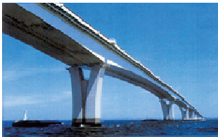
Fig.3 Continuous girder & Y-typed steel piers
