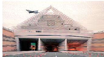
Fig.7 Ukishima Ventilation tower covered with pyramid of pipes
