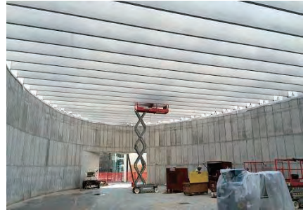
Fig. 2: Precast Roof Joists Spanning Between Cast-in-Place Curved Walls (Photo credit: Guy Nordenson and Associates)
