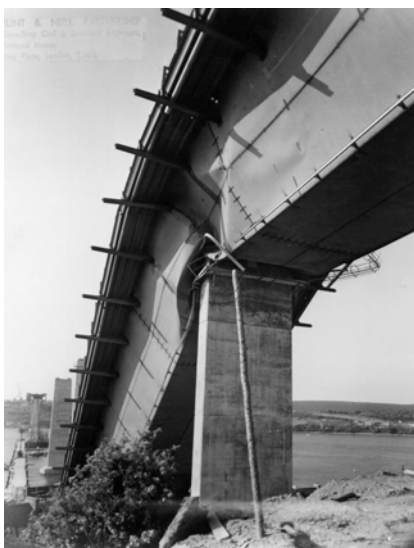
Fig. 1 Milford Haven Bridge, Wales, following the collapse
